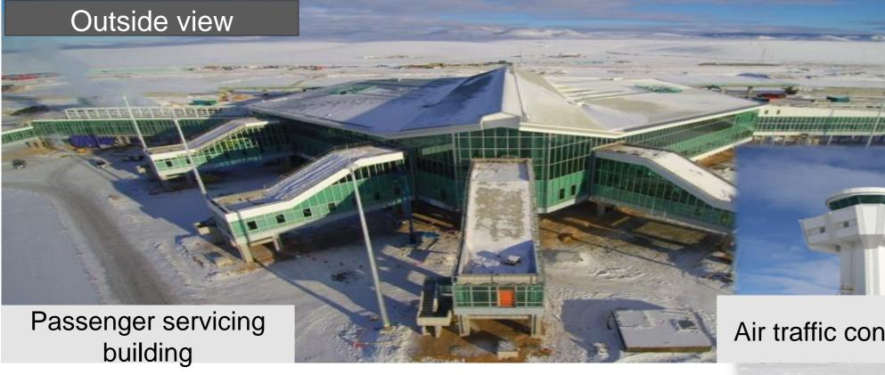
The New Ulaanbaatar International Airport will have capacity for 3 million passengers per annum with passenger servicing terminal with an area of 37,000 sq.m., asphalt runway strips with a length of 3,600 m and 6 aircraft collars with 96,000 sq.m. area.
